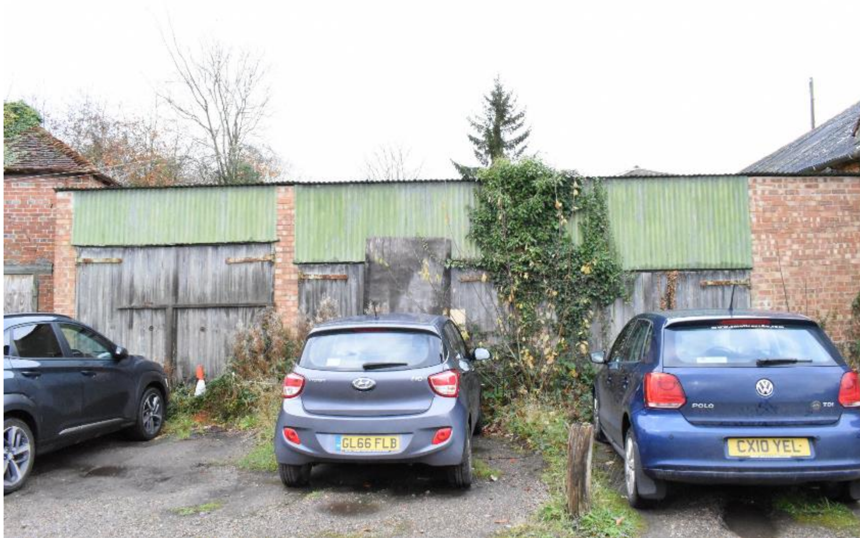
Plate 10: Infill building at southern end of the PDA (facing W)
