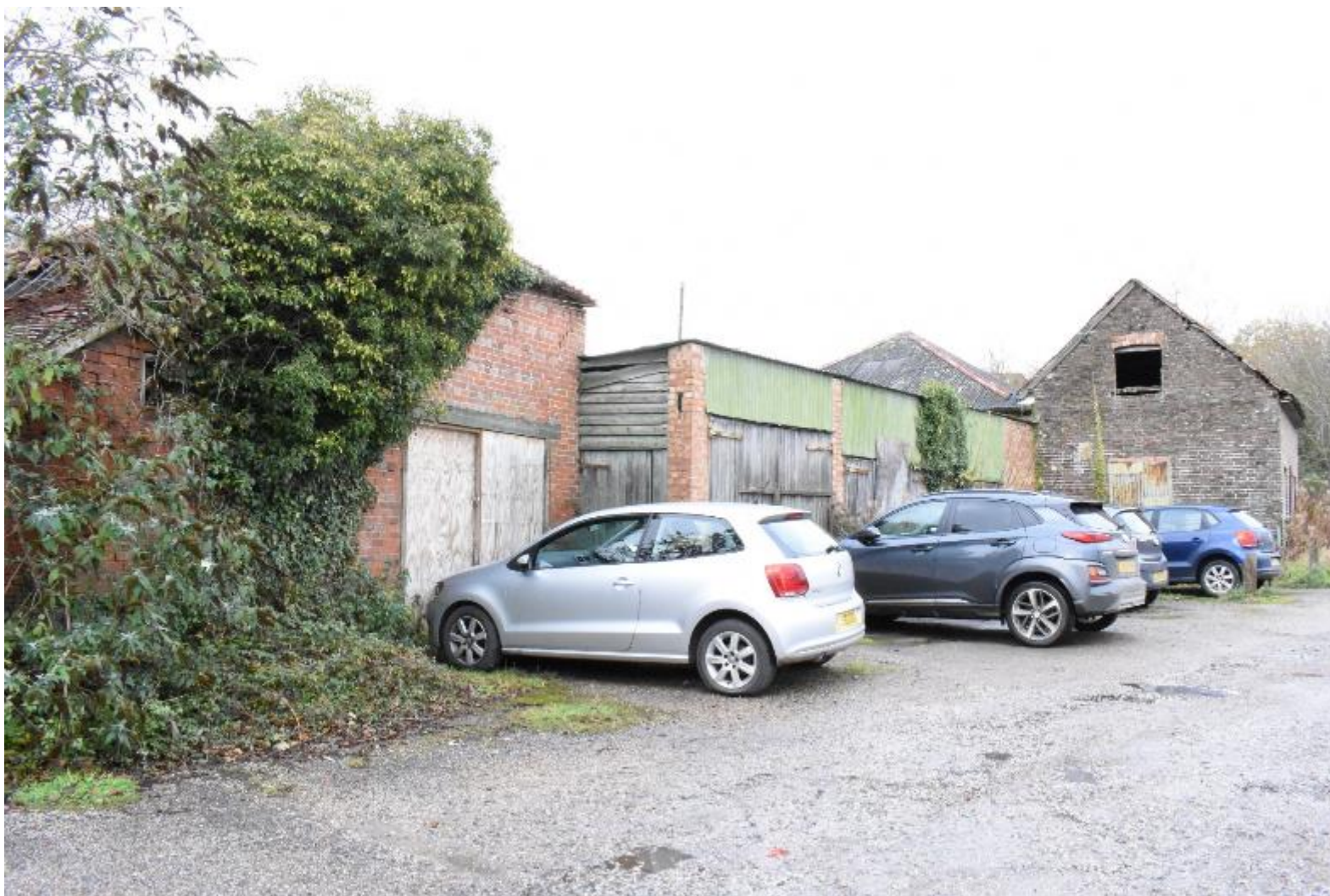
Plate 8: View of the older agricultural buildings from the access road (facing NW).
