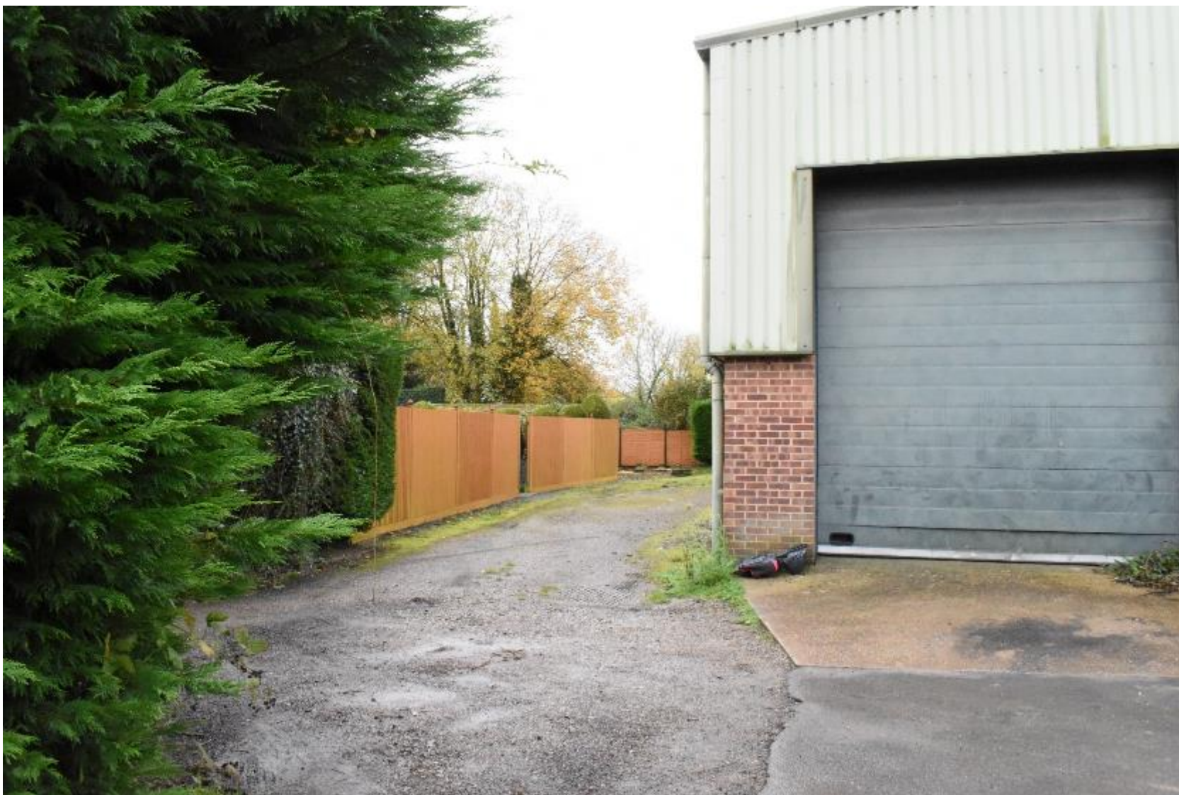
Plate 17: View of the south west boundary at the rear of Old Bassetts Cottages (facing SW)
