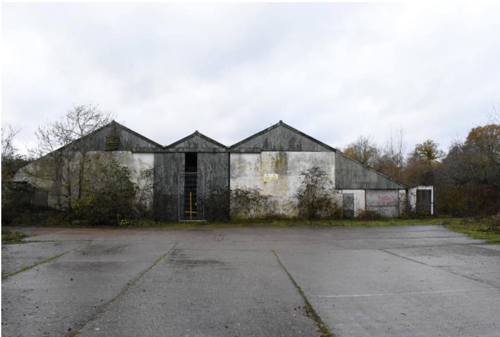
Plate 15: View across the PDA towards the largest agricultural building in the north west part of the PDA (facing SW)
