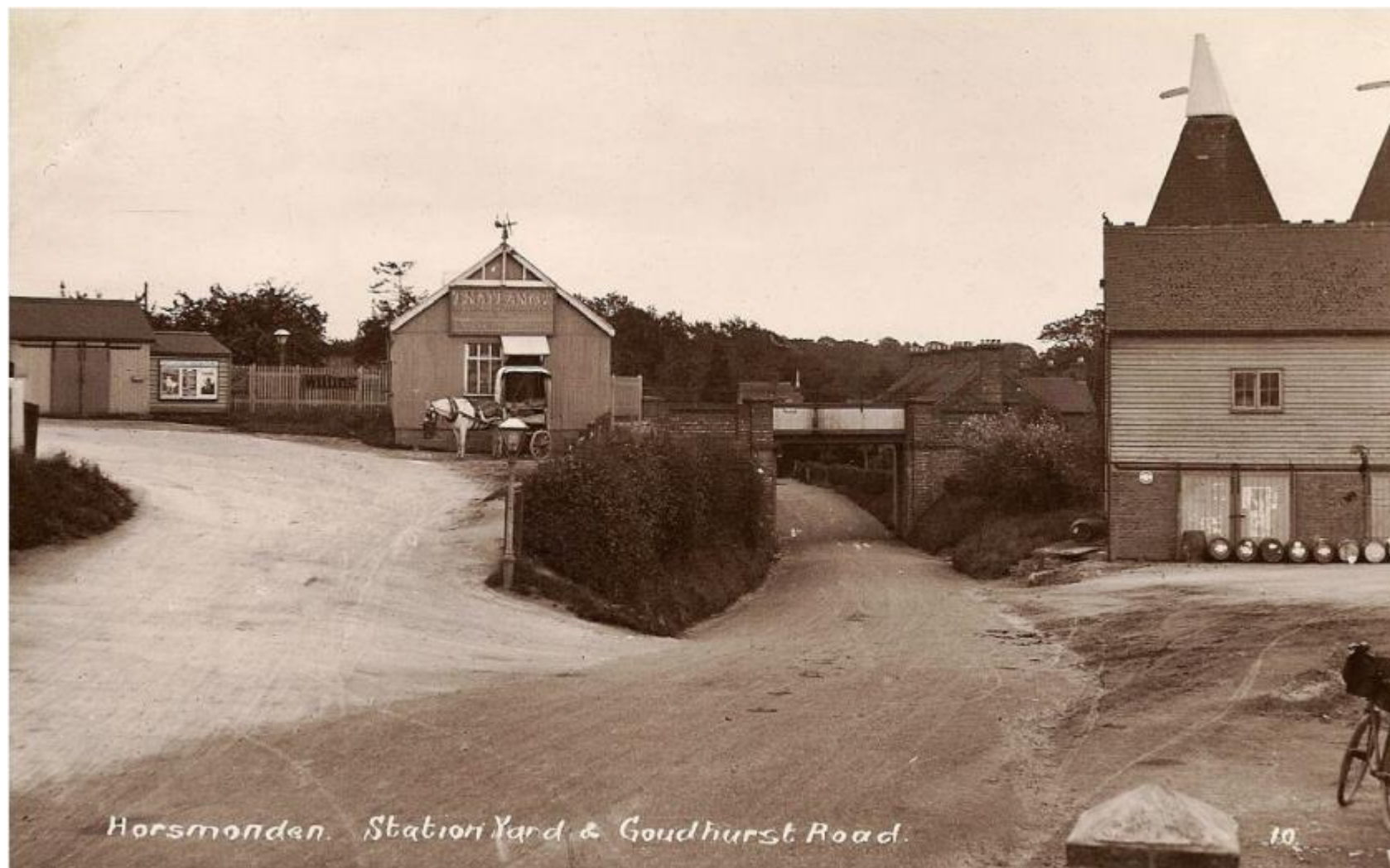
Plate 29: Historical Photo (date unknown) showing the railway bridge over Goudhurst Road. Bassetts Cottages would be just behind the bridge (Horsmonden Village Kent website).
