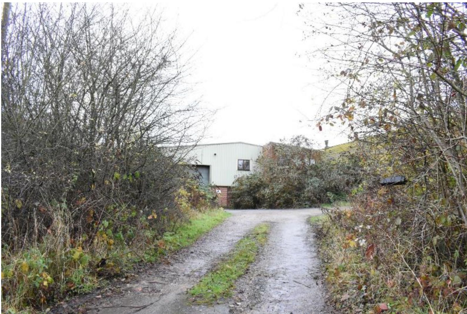
Plate 13: View across the PDA towards the southern modern building. (facing E)
